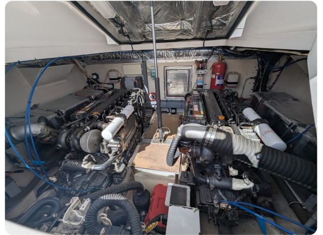
Luhrs 36 Open engine room
