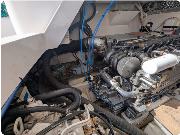
Luhrs 36 Open engine room detail
