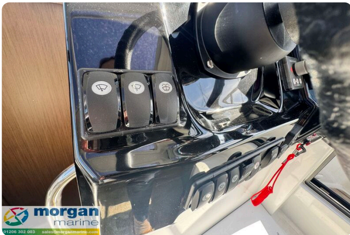
Jeanneau Merry Fisher 895 Offshore - controls
