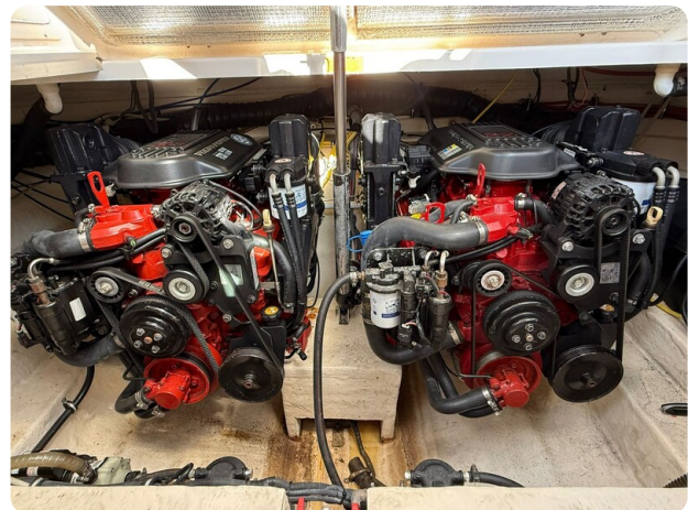
CHAPARRAL SIGNATURE 310 Engine room
