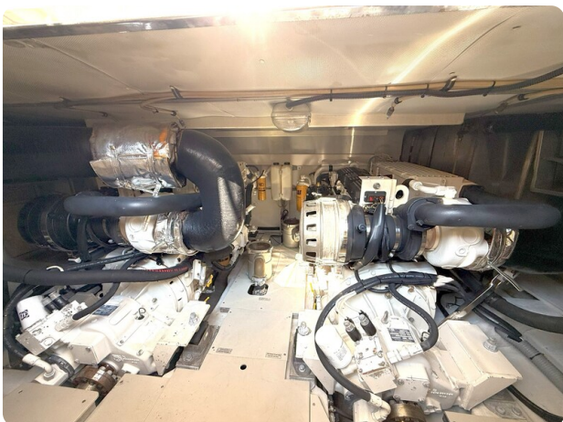
AZIMUT 55 Engine room
