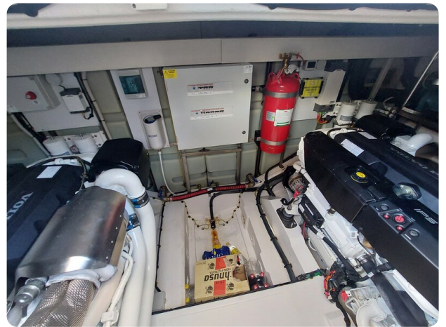
Azimut 53 Fly engine room
